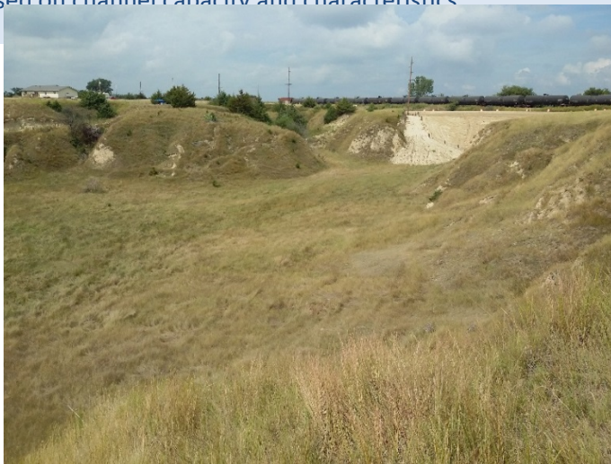
Upper Section of Project Area.
